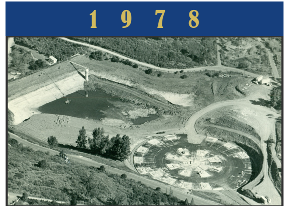
Pechstein Lake is replaced by the covered Pechstein Reservoir.
