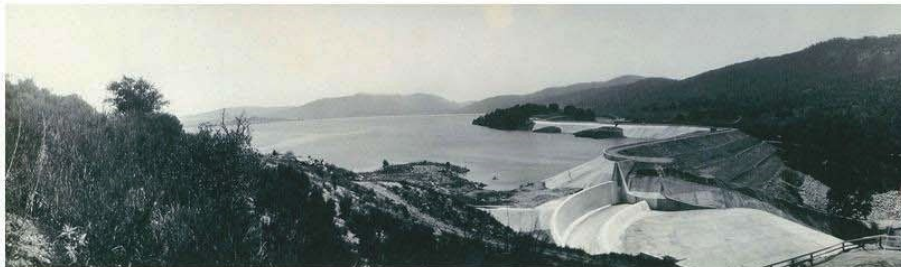
Henshaw Dam April 5, 1928
