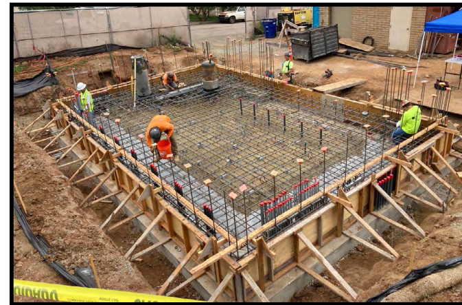
New pump station under construction
