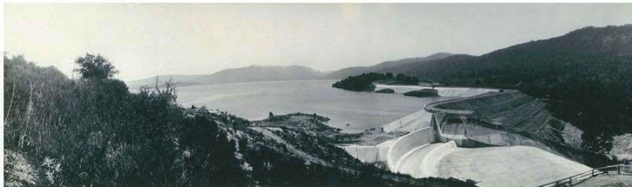
Henshaw Dam April 5, 1928
